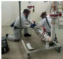
Dust Test Insulation With Bronx Oryza-SIL 650
